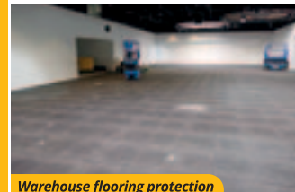
Warehouse flooring protection
